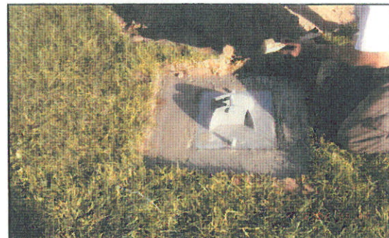
Step 6 Place pillar base in place
