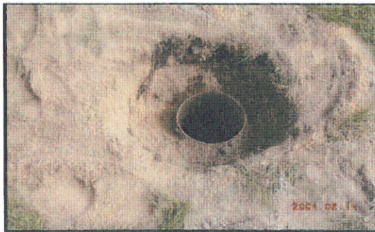
Step 3 Concrete formes for support
