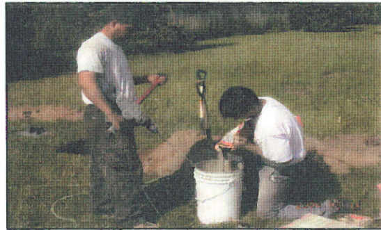
Step 4 Mix concrete
