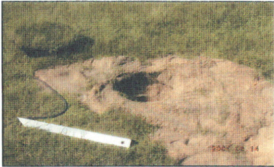
Step 1 Make holes in ground for supports
