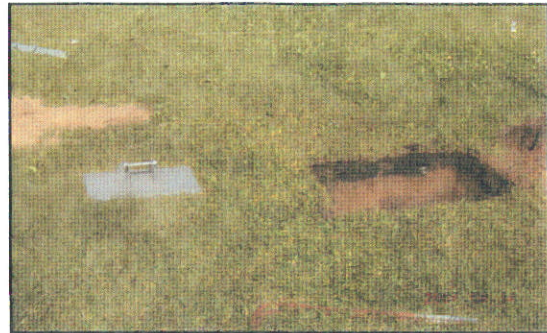
Step 2 Holes for center pillar base
