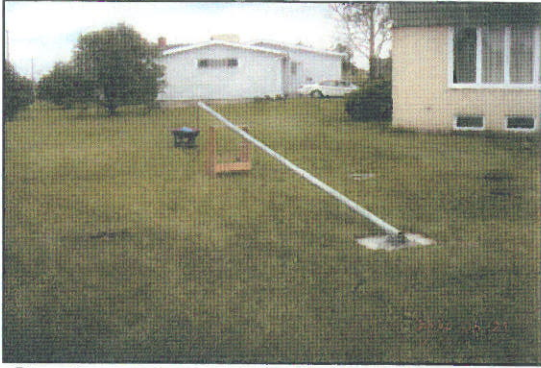
Step 9 Run electrical cable inside Pillar
